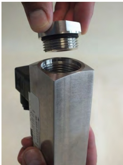
Fig. 35: Remove the process connection (outlet)
