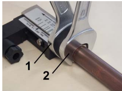
Fig. 11: Screw in the device
